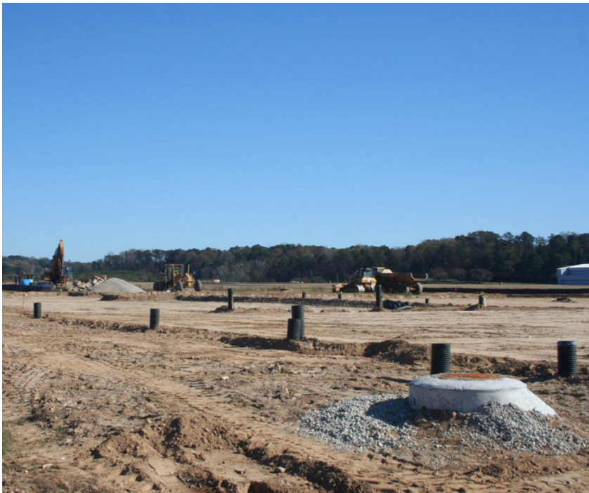
Image of construction happening along Sandy Creek Drive where new tenants are coming in.
